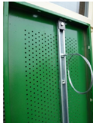
Internal Unistrut bar and fixings
